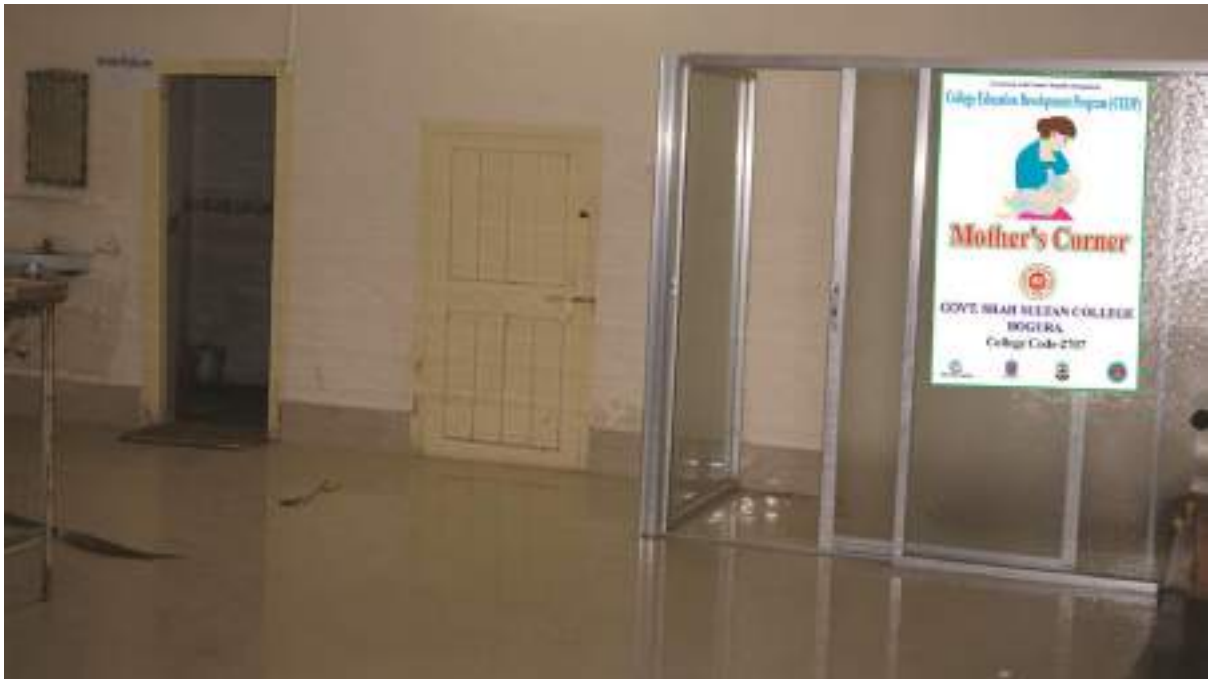
Female Common Room and Mother's Corner Refurbished & Renovated by CEDP
