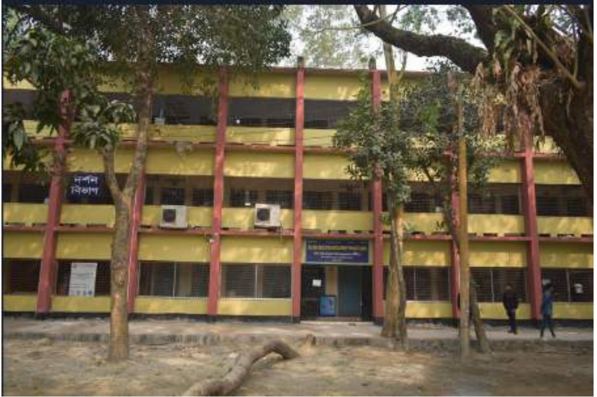
After Refurbish & Renovation Academic Building-05 & CEDP Office and ICT Lab
